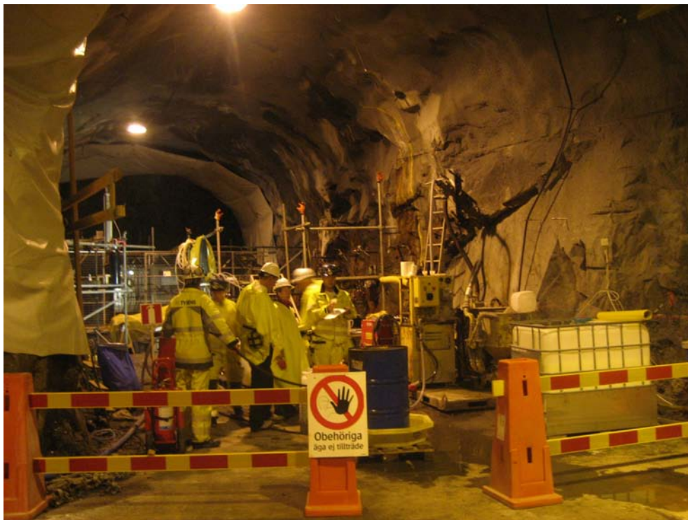
Figure 4-1. Grouting tests in Äspö HRL, September 2007.
