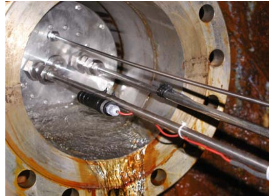
Installation of first model canister assembly
